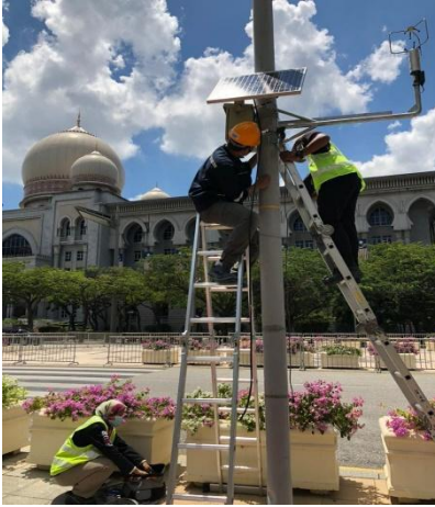
(a) Ultrasonic anemometer being installed in Precinct 3 (UKM01)
