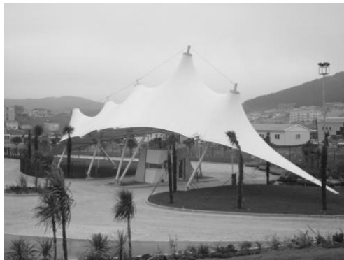
Figure 1: Tensioned Fabric Structure
